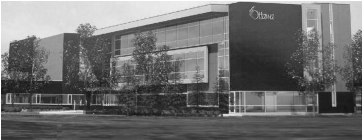
Figure 3: New Ottawa City Archives Building
