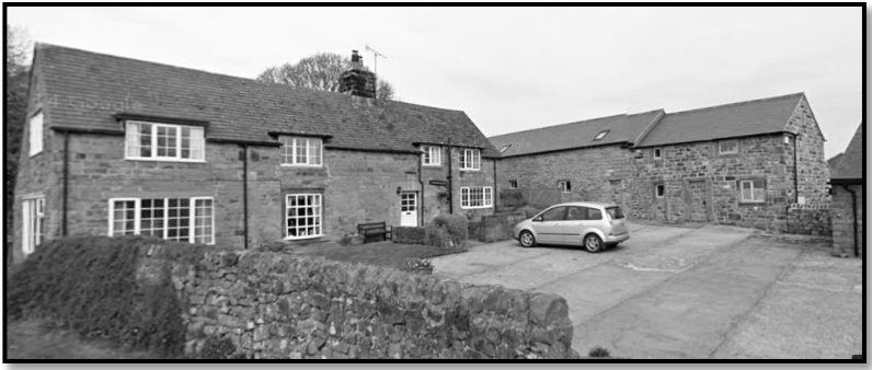
Figure 5: Hill Top Farm, Ashover
