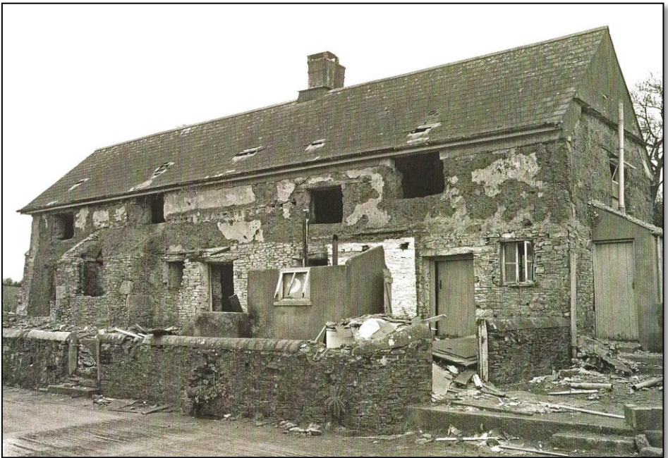
Figure 4: Shop farmhouse during demolition. Notice the pigeon holes between the middle two windows on the second floor . . .
